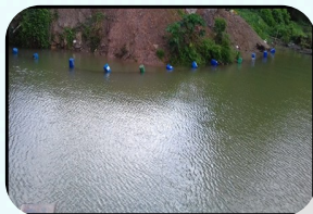
Installation of Silt Curtain at riverside
