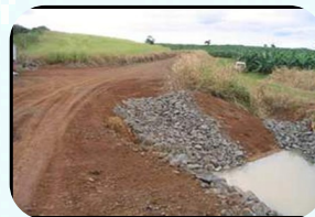
Implementation of Silt Trap
