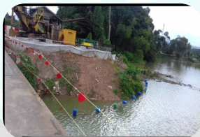
Installation of Silt Fence at the slope
